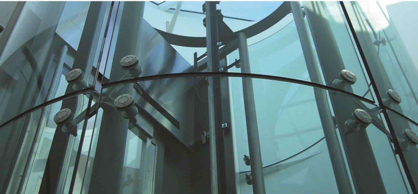
A fascinating design element that enhances any facade. Whether in straight-lined or segmented facades, or circular configurations with curved glazing, Gentry Spider Fittings meet requirements of functionality and aesthetic elegance.
